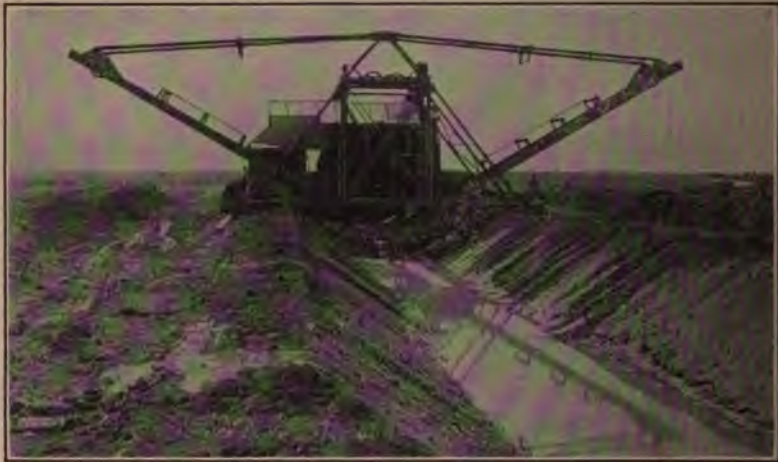
Austin Templet Excavator with Narrow Bottom Frame.
